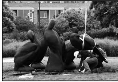
Installation of these 400- to 700-pound sculptures took ingenuity, patience, and skill. Photos © Rebecca Miller
