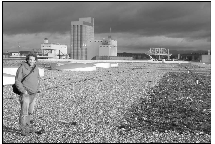
Stephan Brenneisen on the new Stucki Shopping Center ecoroof in Basel, Switzerland. This ecoroof incorporates cobble and gravel substrates meant to mimic floodplain or river terrace habitats. © Jim Labbe
