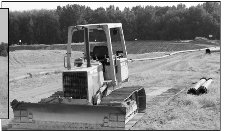
Port of Portland placing contaminated sediment on West Hayden Island. © Bob Sallinger
