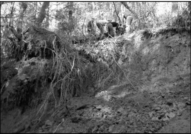
Constructing a detour around trail section wiped out by a recent landslide. © Tom Costello
