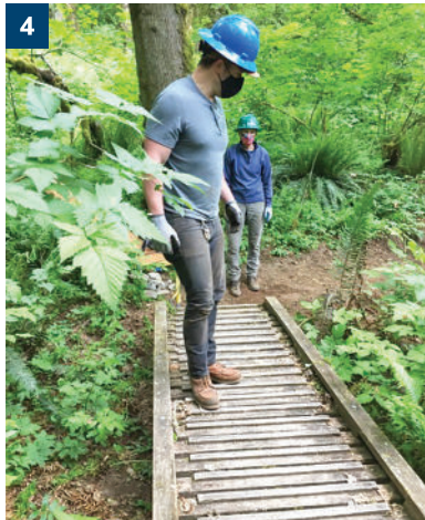
4 Braden and Geri (TKO advisor) check for levelness and even distribution. After installing risers and securing the repurposed bridge, it was good to go.
